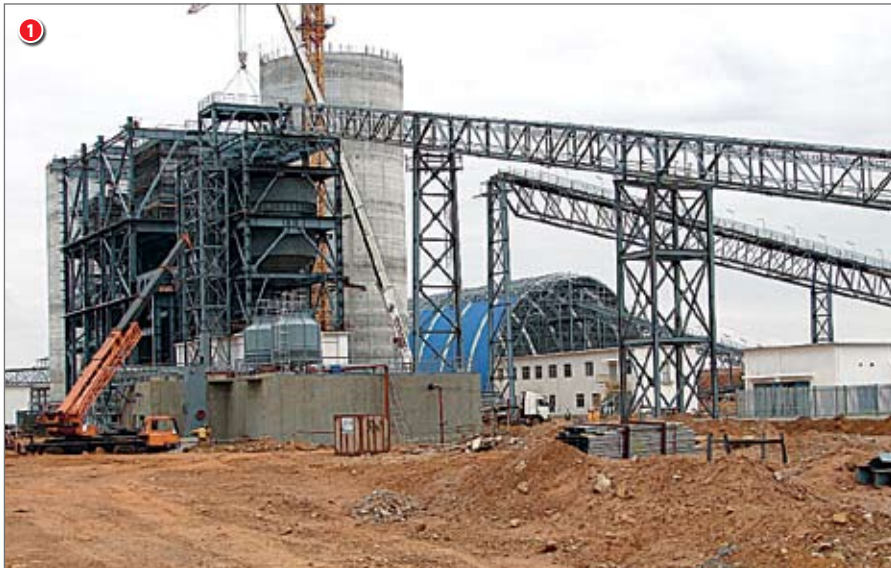
1 Lafarge's Randfontein grinding plant under construction
