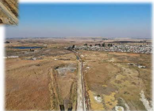
Pipeline to Ergo plant
